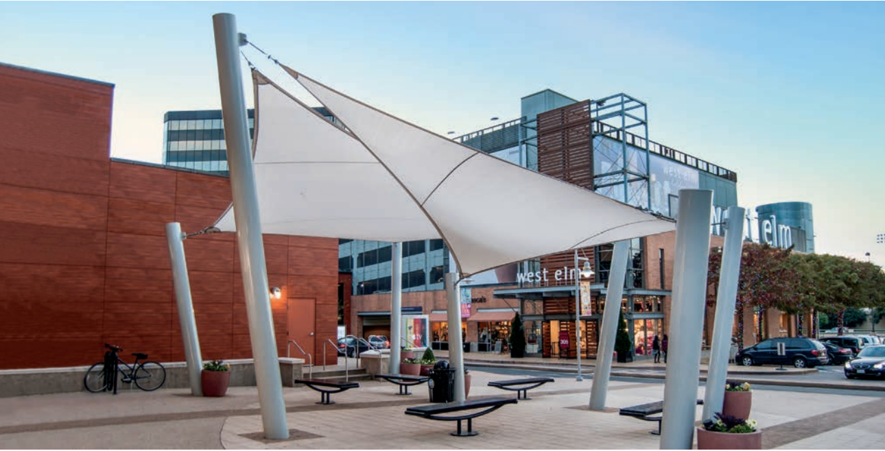
Mockingbird Station Dallas, Texas
