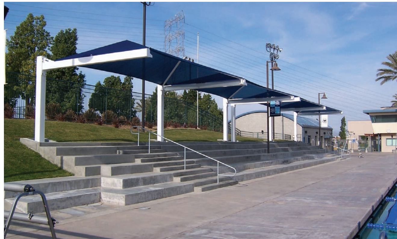
single tri-truss cantilever joined
