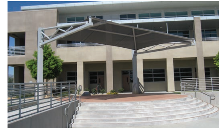
single tri-truss cantilever
