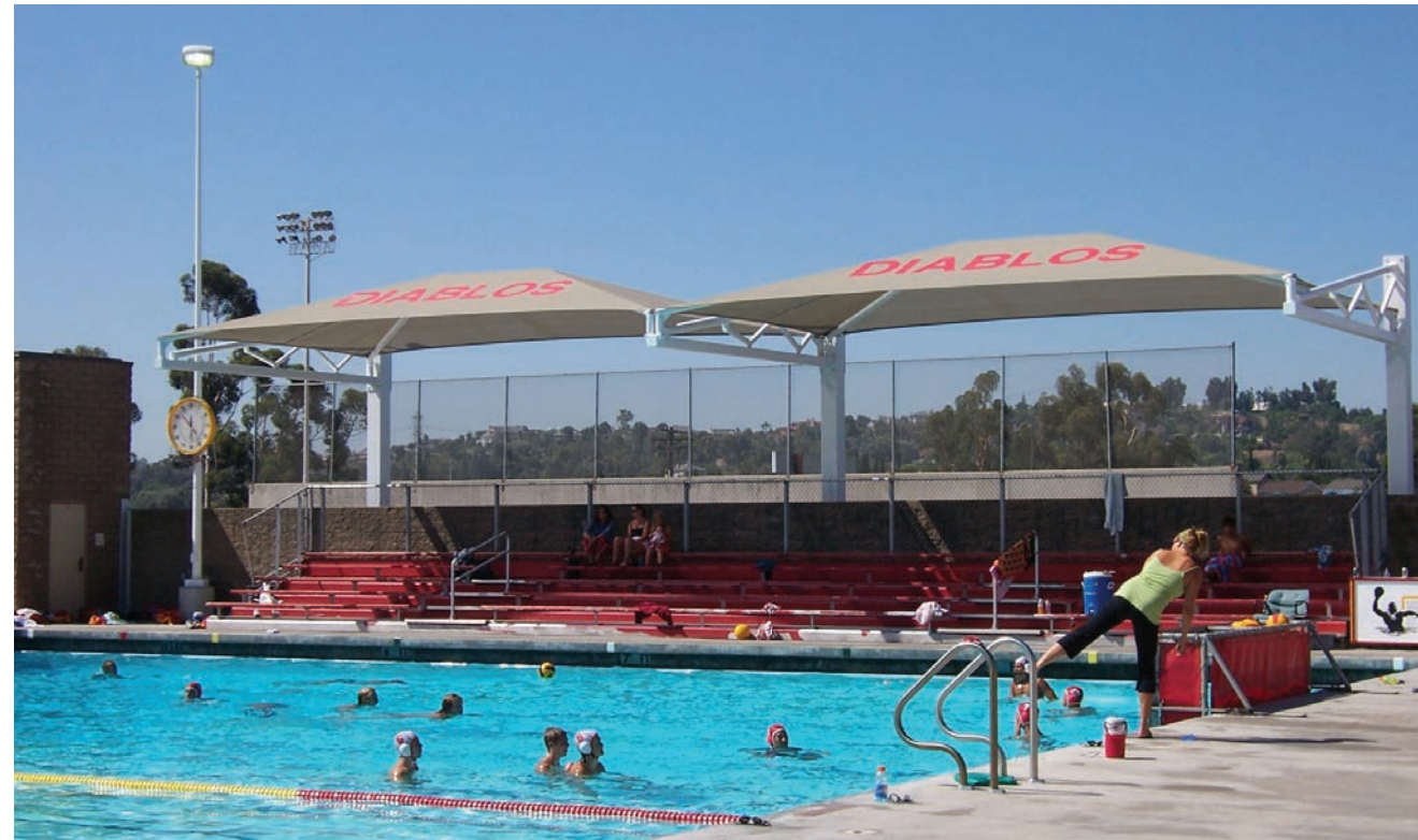
single tri-truss cantilever
